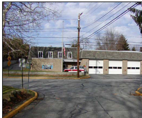
Broad Street Fire Station
