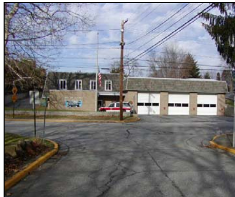
Broad Street Fire Station
